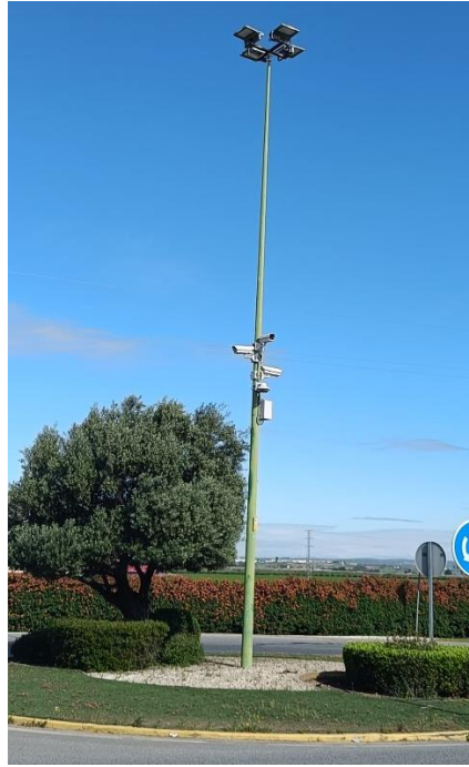
LOCATION 6.1: AFTER THE IMPLEMENTATION
